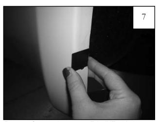
Remove flare and center a Tab (MT1-0002) over each of the four locations marked in Step 5.
