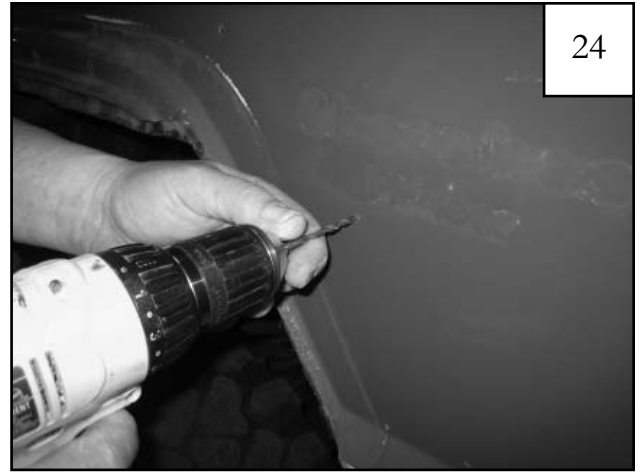
Drill marks with a 3/16" bit.
